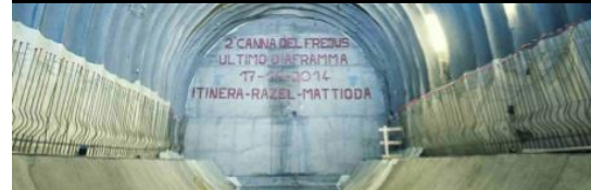
FREJUS: from the historical tunnel (1871) to nowadays tunnel
